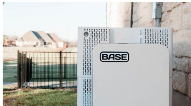
Often paired with rooftop solar panels, residential battery storage systems can provide backup power during outages, keeping essential equipment like lights, refrigerators and medical devices running.
